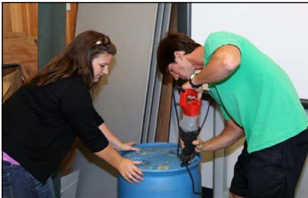
Educators Lydia Courtright and Jim Gould work to cut off the top of a recycled barrel. Once the lid was removed, the barrel was washed out and window screening was placed over the opening for rainwater to pass through (courtesy of [jennettespier.net/Daryl Law](http://jennettespier.net/DarylLaw) photo)
